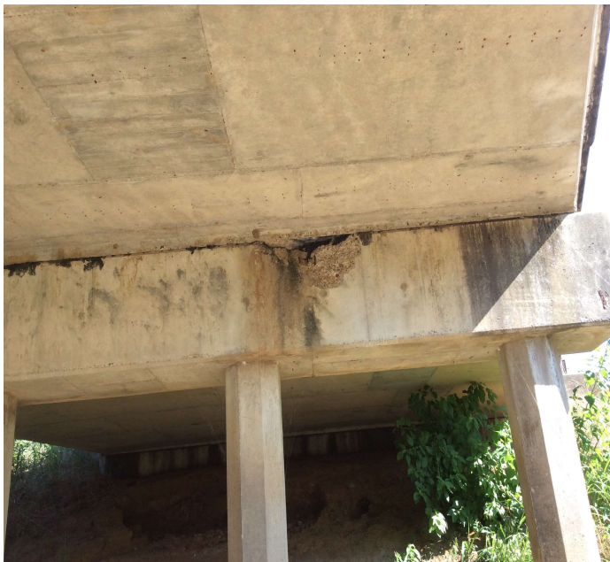
PHOTO 1 Description Spall cap bent 2 Spalls on cap faces bent 2, 3, 4, 5, & 6
