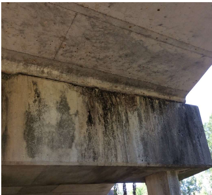
PHOTO 4 Description Spall bent 5 cap north face
