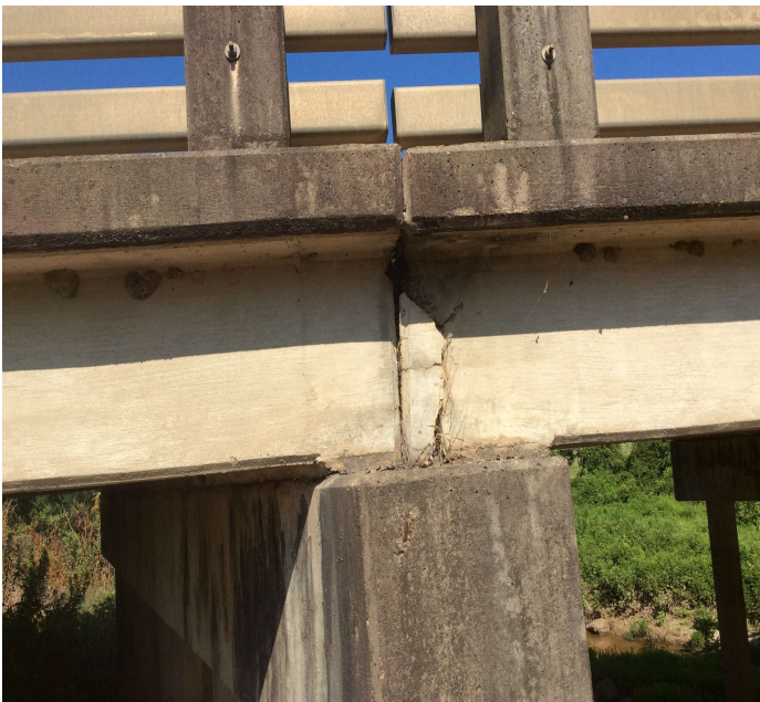
PHOTO 1 Description Bent 5 left side corner of slab spall
