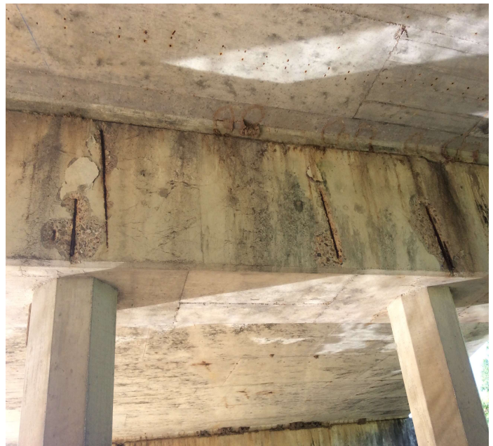
PHOTO 2 Description Bent 3 rebar exposed
