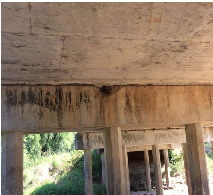
PHOTO 3 Description Bent 4 cap spall south face
